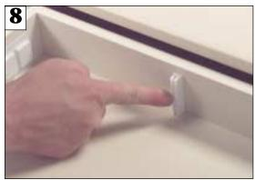
8. Attach the holder to the back of the drawer where you made a mark for the next grooved strip.
