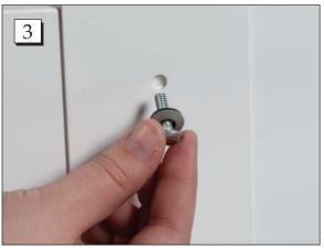
**Step 3.** Place the bolt and washer thru the top hole of the hanger and box.
