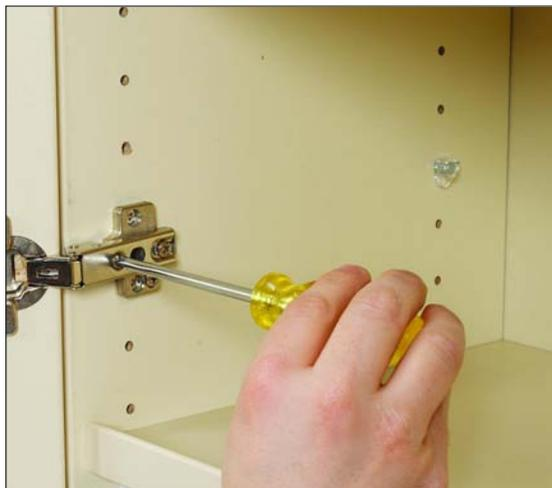
**The left adjustment screw provides depth adjustment:**
