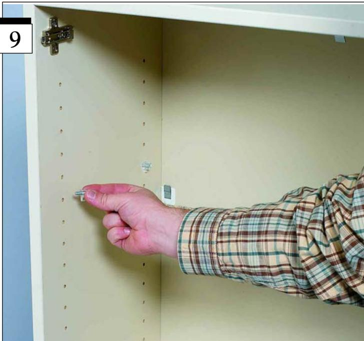
Decide the positioning of your shelf. The shelf is adjustable in 1/4" (32 mm) increments. Insert the clear plastic shelf pins in the back holes at your desired height. Once the back shelf pins are in place insert shelf pins into the front shelf holes at the same height as the back pins.
