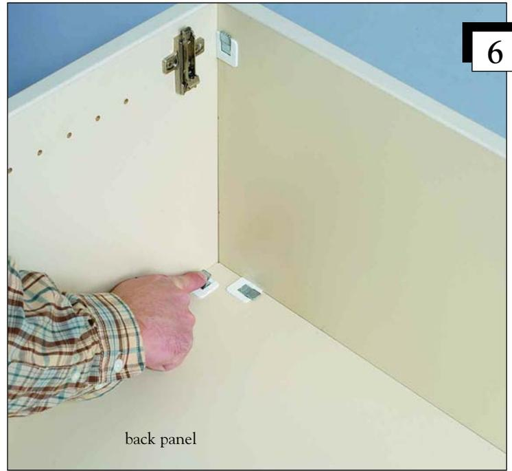
Push the panels together and press the fitting toggles down to secure.
