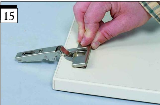
Once hinges are in place and flush against doors, press down on the screw cover plates to secure hinges to doors.
