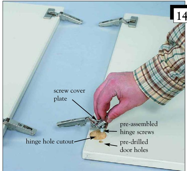
Begin by laying the doors flat on the ground with the hinge hole cutouts (inside of doors) facing up. With screw cover plate lifted, insert pre-assembled hinge screws into the pre-drilled door holes. There are two latches per door.
