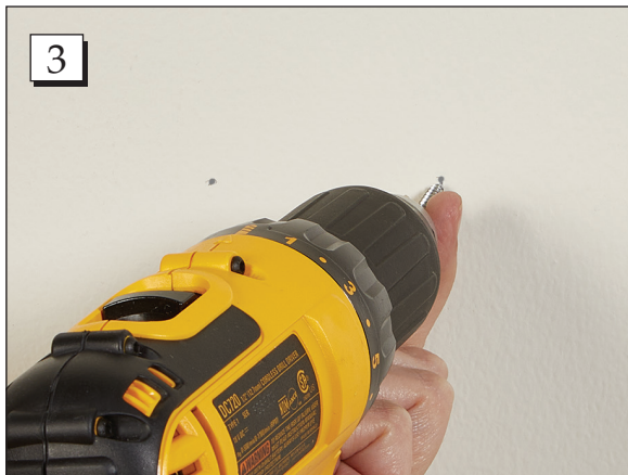
Step 3. Drive a screw into each marked hole.
