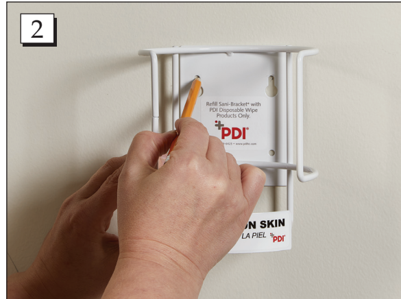
Step 2. Use a pencil to mark the screw holes.
