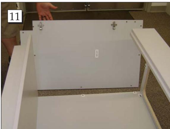
**Step 11.** Attach the left side by aligning the pre-drilled holes with the connection fittings in the back, top and bottom panels.
