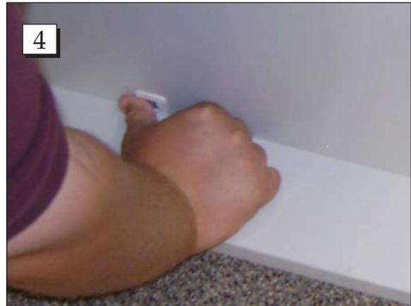
**Step 4.** Once together, press the fitting toggles down to secure.
