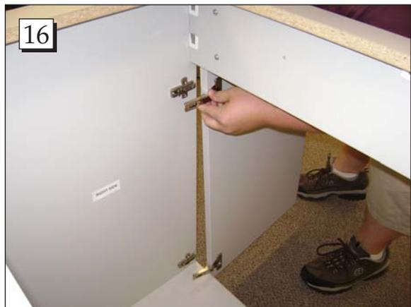
**Step 16.** Doors are ready to be attached. Position the left door onto the side of the cabinet unit. The hinges should align with pre-installed hinge plates mounted inside of the unit.
